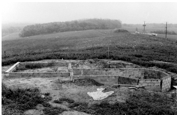
Nearly finished foundation for the Oscar Mayer Observatory. Photo from Steve Bracker's collection, 1960.
