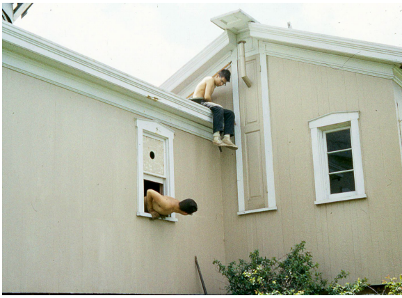
Preparing the Student Observatory for the move. John Rouse is leaning out the window. The unknown boy on top is sawing into the eaves of the building, the tip of the saw just visible under his left sneaker. An iron breaker bar can be seen leaning against the building at lower center. Taking most of two summers, the prep and the move created many blisters and indelible memories for the kids involved. Photo from Eric Thiede's collection, July, 1960.
